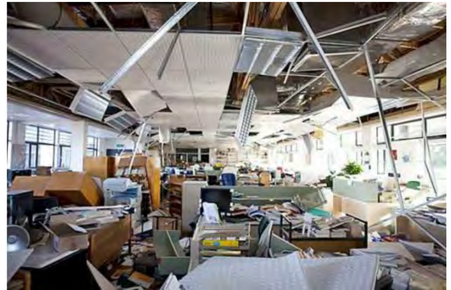
Ceiling damage in the 2011 Christchurch Earthquake in New Zealand
