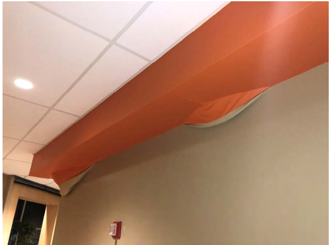
Water damage in 2018 Anchorage Earthquake
