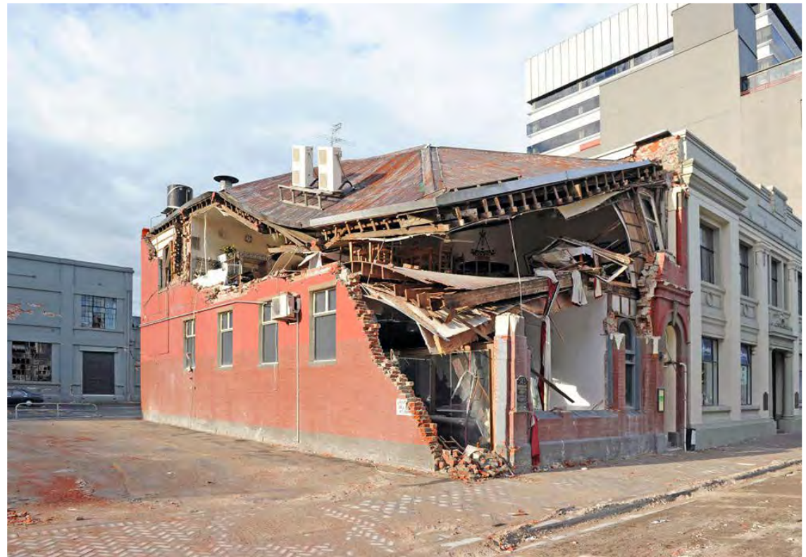
URM Building Damage in 2011 Christchurch, NZ Earthquake
