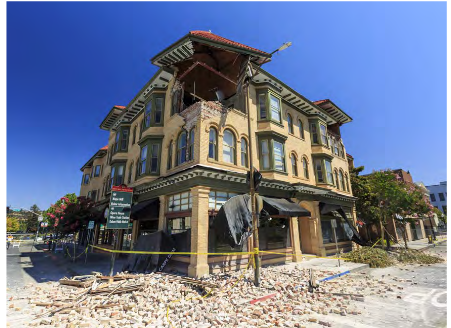
URM Building Damage in 2014 Napa Earthquake
