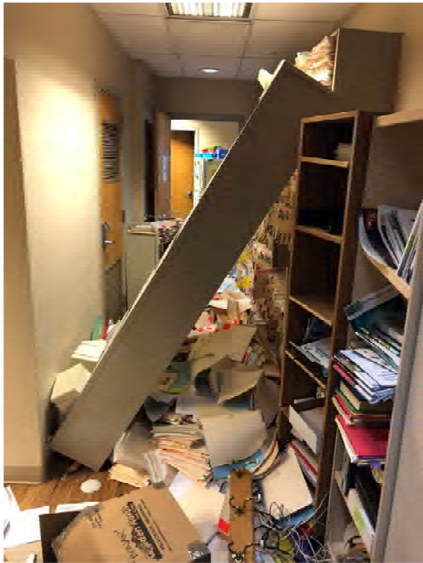
Overturned Contents in 2018 Anchorage Earthquake
