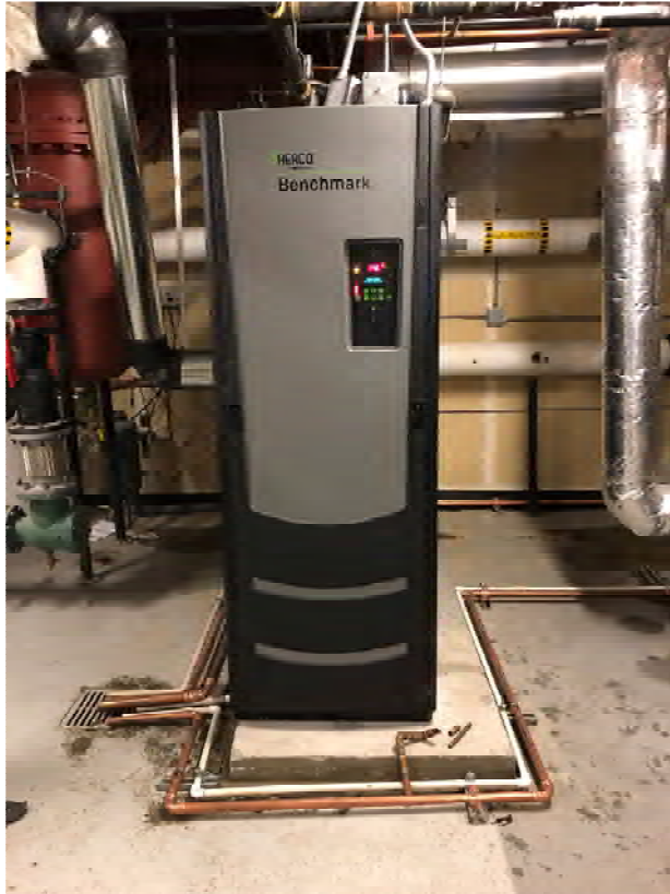
Unanchored boiler shifted and broke natural gas line in 2018 Anchorage Earthquake
