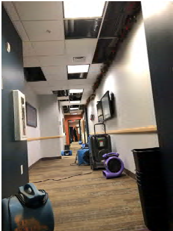
Water damage from domestic water line break in 2018 Anchorage Earthquake
