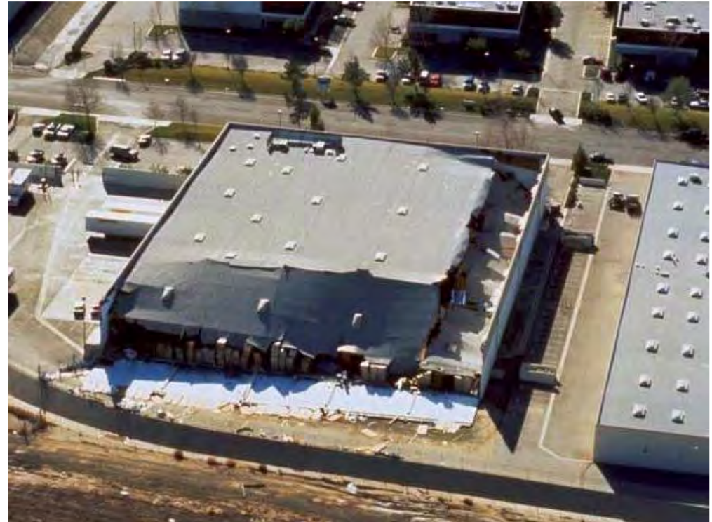
Wall Anchorage Failure in 1994 Northridge Earthquake
