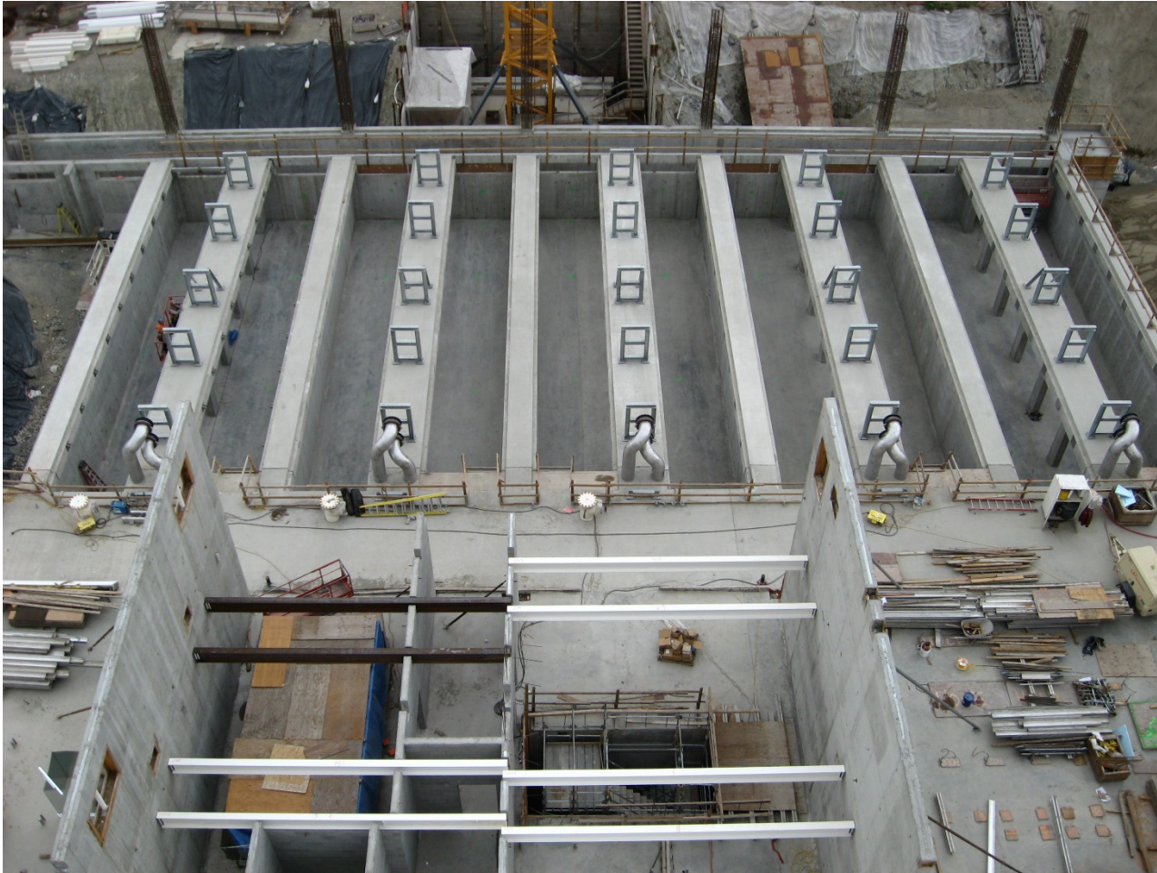
Membrane Tanks – 10 Tanks - 70' Long x 28' Wide x 14' Deep
